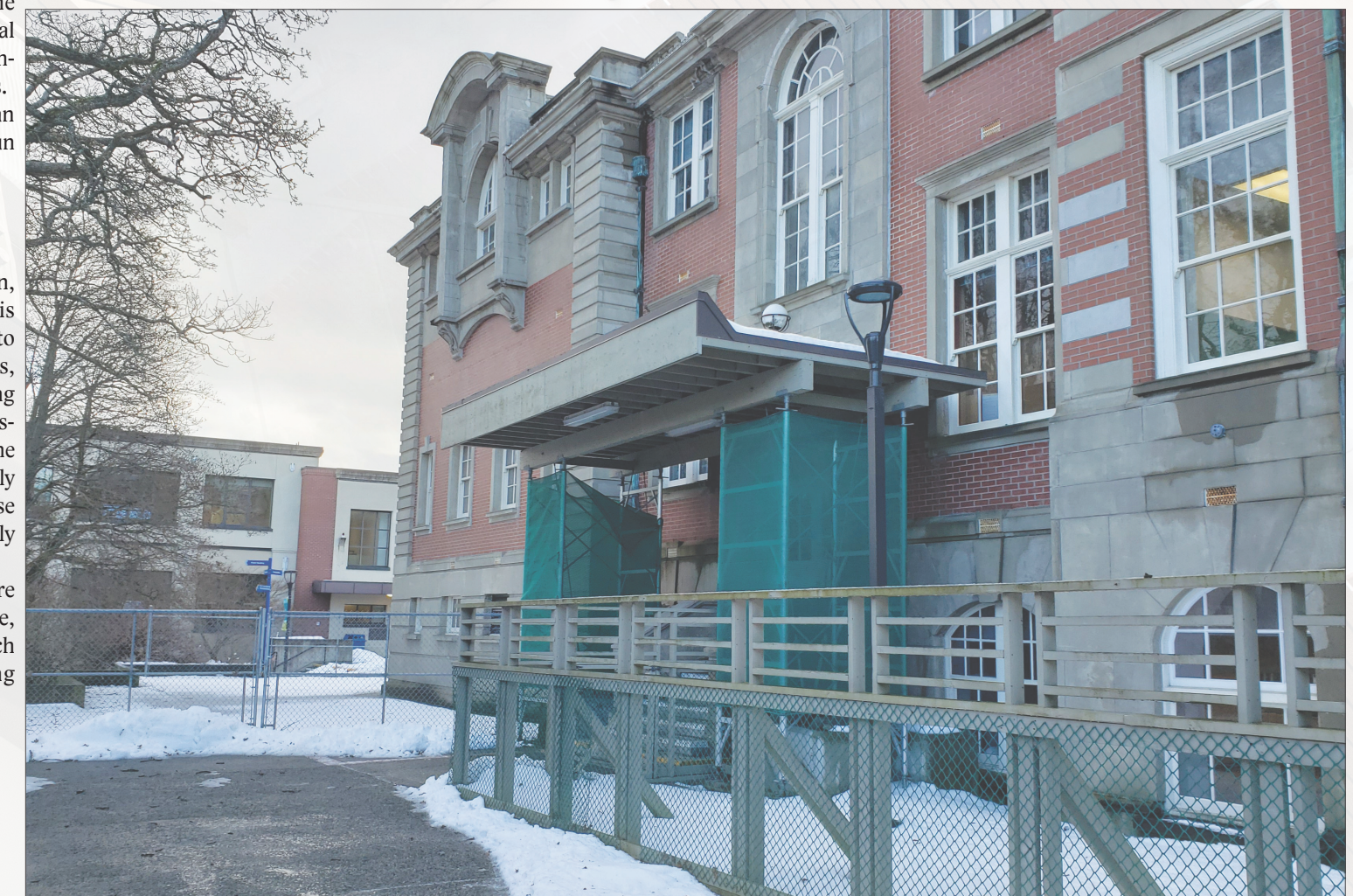
The exterior of the Young Building, located at the Lansdowne campus.
